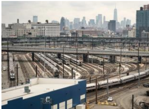
Sunnyside Yard under Amtrak ownership
