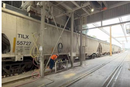
Port of St. Louis grain unloading facility.
