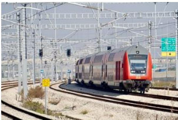
Modern multi-track railway infrastructure – Herzliya Station.
