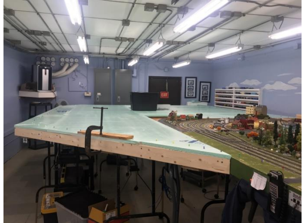
August 29: Oops, we missed a few spots in the foam gluing process. Photo by Ken Howard
