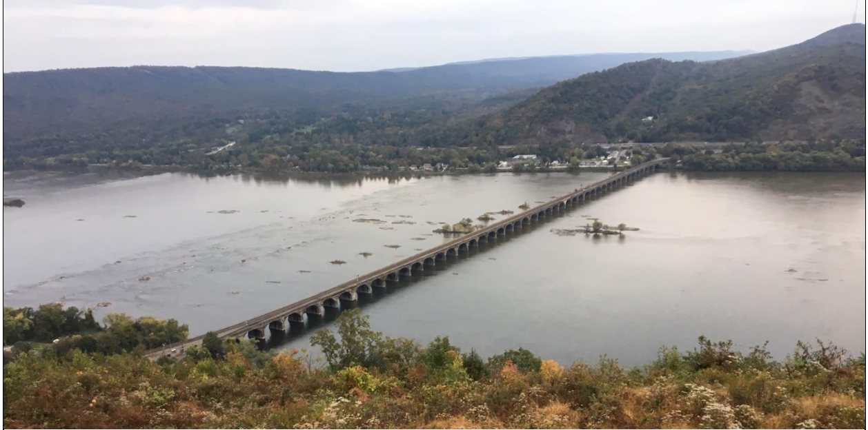
View of the Rockville Bridge across the Susquehanna River from Marysville, PA.
