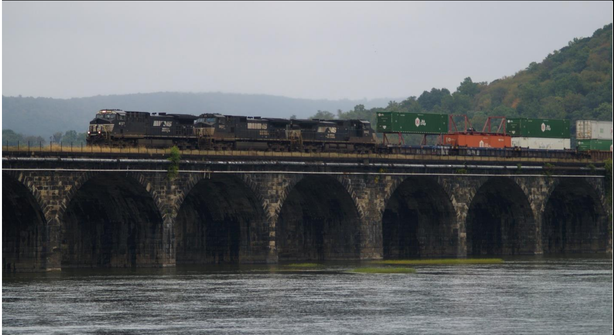
Norfolk Southern stack train crossing the Susquehanna River on the Rockville Bridge in Marysville, PA. The Rockville Bridge was completed in 1902 by the Pennsylvania Railroad and remains the longest (3,820 feet) stone masonry arch railroad viaduct in the world.
